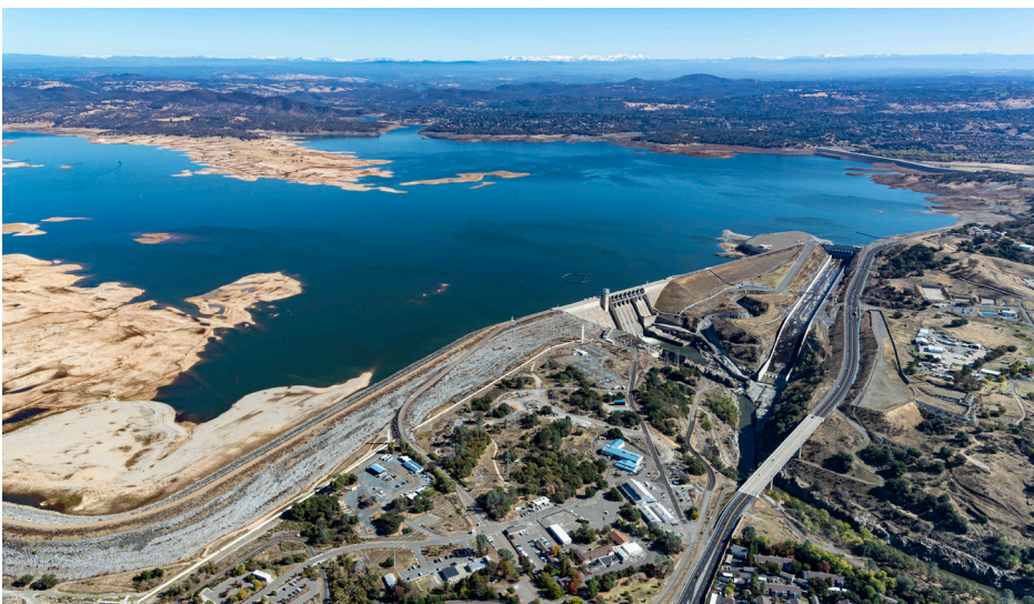
This aerial view shows low water conditions at Folsom Dam in Sacramento County, when on this date, the storage was 309,573 reservoir acre-feet, which is 32 percent of the lake’s total capacity. Photo taken October 28, 2021. Caption and photo credit: California Department of Water Resources/Andrew Innerarity
