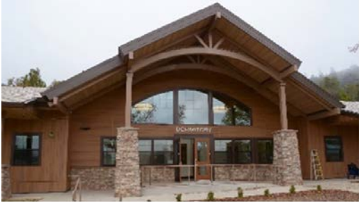
Completed Placer Center dormitory building.
