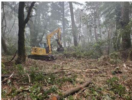
Figure 33 Grant to the to the Marin Municipal Water District to implement vegetation management projects identified in the Biodiversity, Fire, and Fuels Integrated Plan (BFFIP) in the Mount Tamalpais Watershed, and to reduce ladder fuels in the Marin County Parks Blithedale Summit Preserve.
