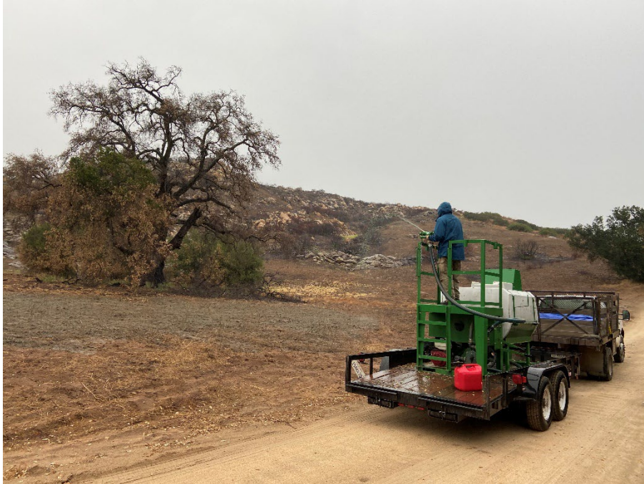
Figure 7 Hydroseeding at Canada de San Vincente Ecological Reserve
